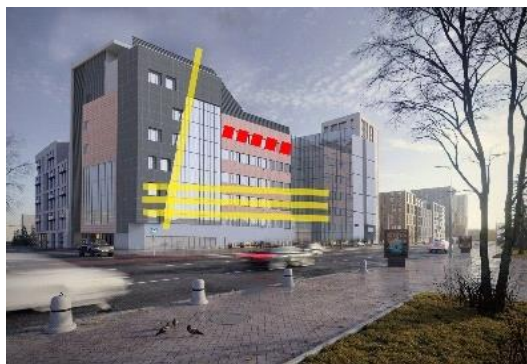
Figure 5.4. View of Jam Hospital
