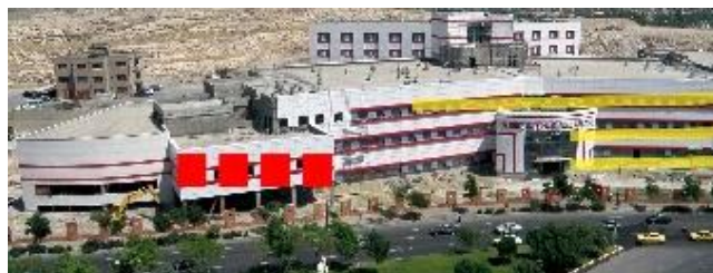
Figure 5.11. View of Vali Asr Hospital in Tabriz
