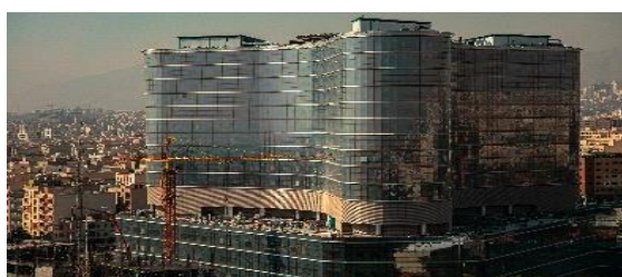
Figure 5.10. View of Mehdi Clinic Hospital
